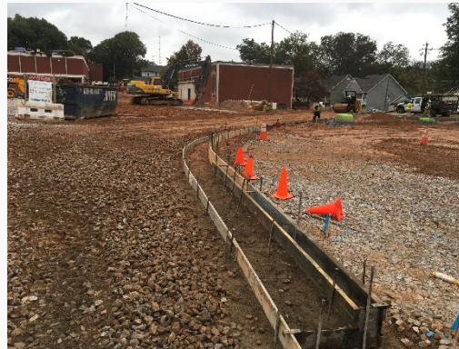
Installation of Curb and Gutter
