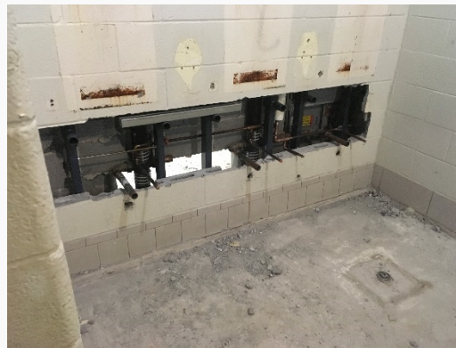
Renovation Framing and MEP Rough
